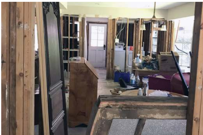
Gutted home in the aftermath of Hurricane Harvey. Image courtesy of Anthropocene Alliance.
