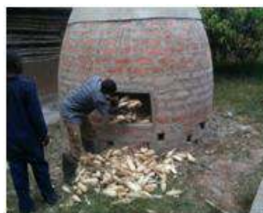
Figure 11: ISSB Granary at a Medium Farm
